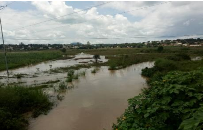
Photo/Picture 13. Inondations derrière CAMI Toyota. Flooding behind CAMI Toyota.
